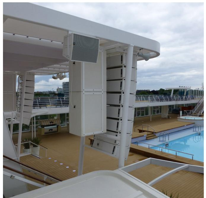
This space required three separate, switchable sound systems: a main Left/Right O-Line hang, with subwoofer support for band set-up; an additional cinema surround, for when the room reverts to movie mode and an acoustic control system to set the venue for different reverberation times — for instance when a string quartet or piano soloist are performing.
